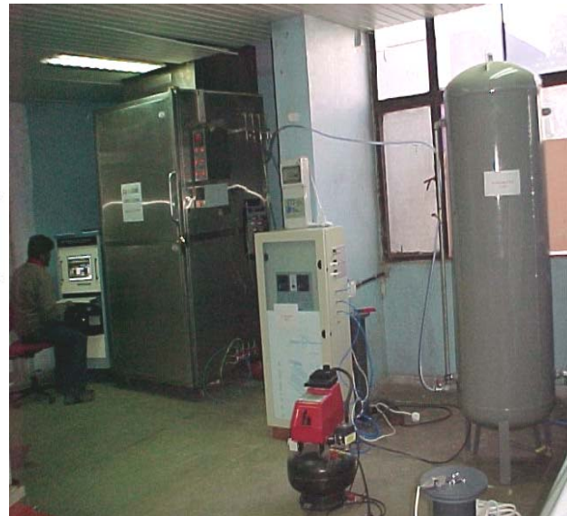
Fig 2: CA chamber along N 2 Generator
